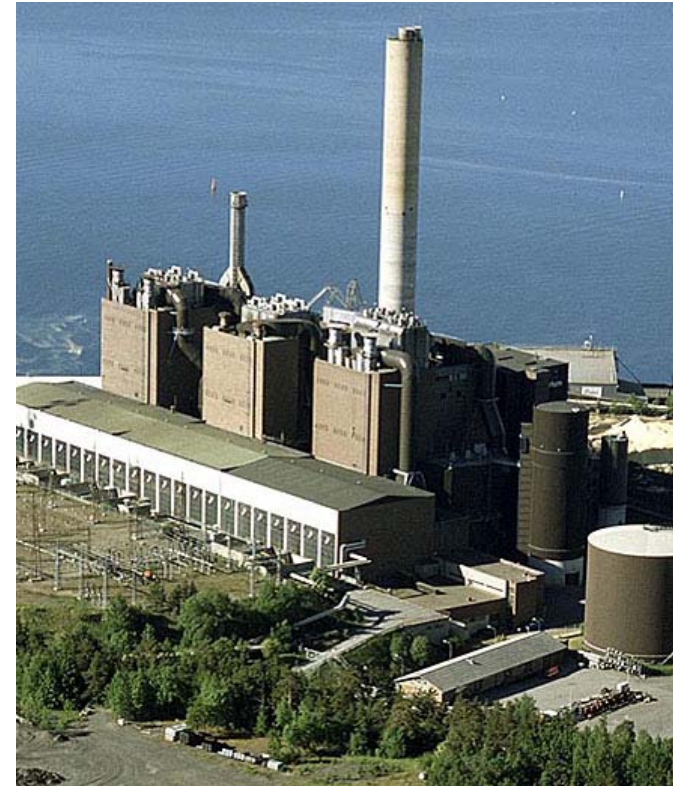
Naantali CHP plant provides heat for the city of Turku
